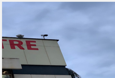
CCTV camera installation complete (bottom to top)
