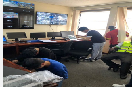
Traffic control room server and monitor installation
